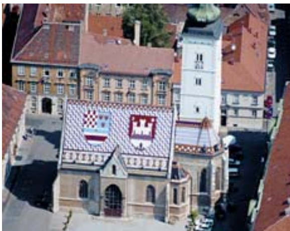
St. Mark's Church – Zagreb
